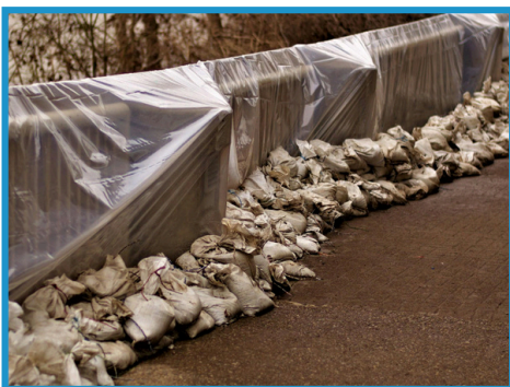
Deployment of traditional sandbags
