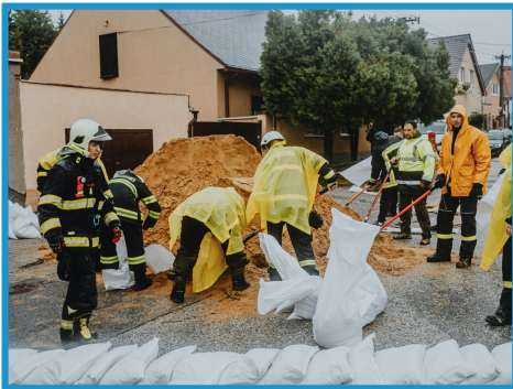
Preparation of traditional sandbags
